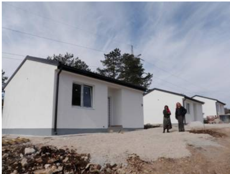
Trebinje Municipality, a total of 4 new housing units built
